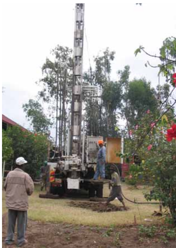
The much larger drill rig did the job
